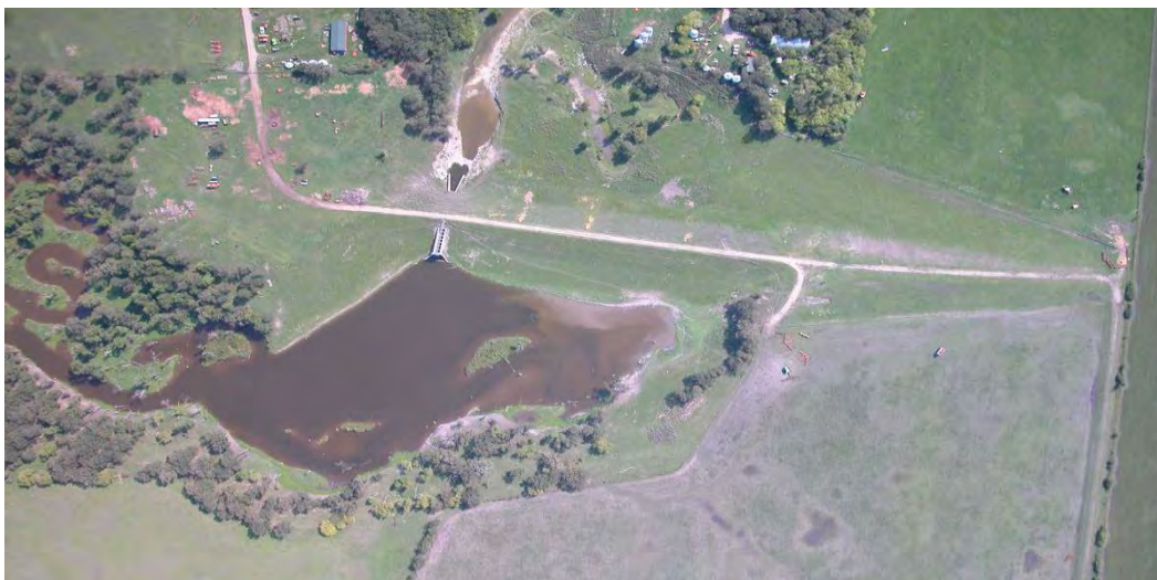
Aerial view of Schirrick Dam looking south
