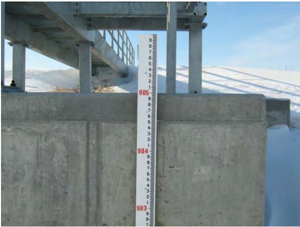
Typical staff gage at structure
