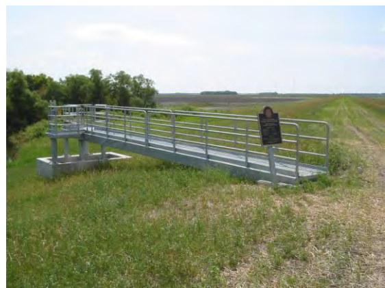
Principal Outlet Structure
