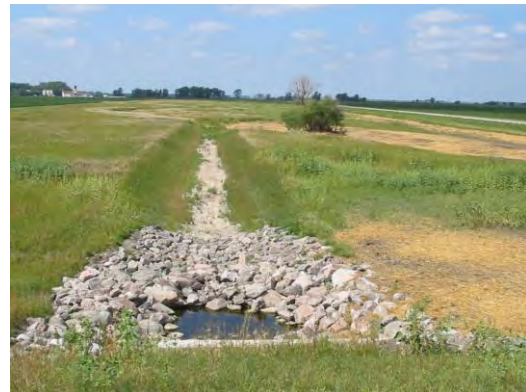
Principal Outlet structure looking west
