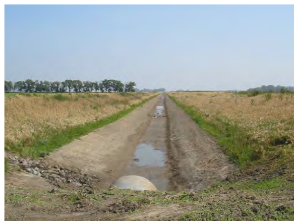
Completed ditch section
