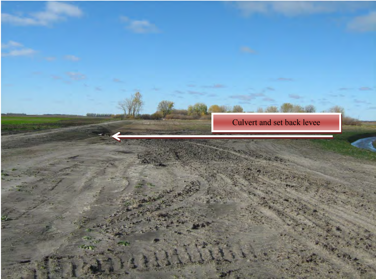
Set back levee and culvert for field drainage
