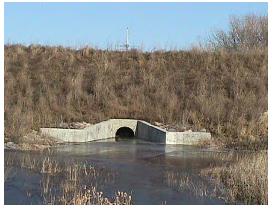
Principal outlet structure (outlet end)
