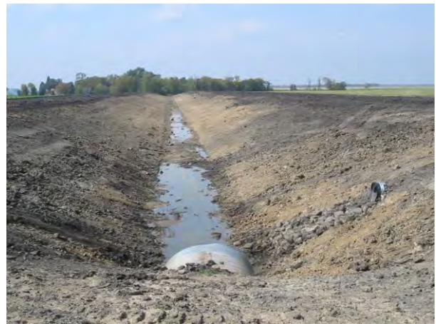
Recent excavation near outlet of ditch
