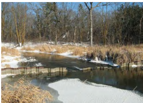
Stoplog sheet pile dam
