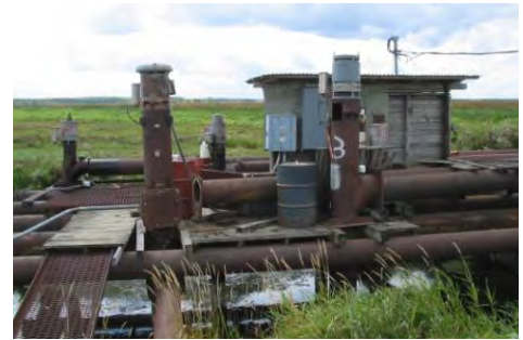
Typical pumping station
