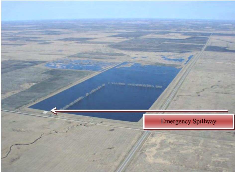
Aerial view of Parnell Impoundment
