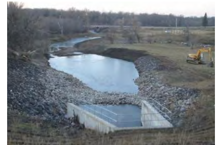
Looking downstream from outlet structure
