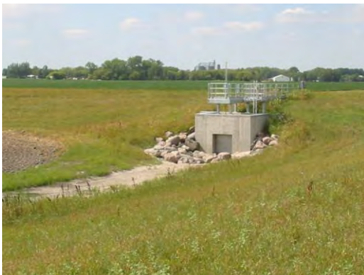
Principal Outlet Structure
