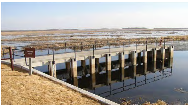
Stoplog Outlet Structure
