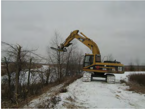
Mechanical brushing along alignment
