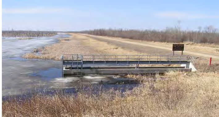
North Pool - Gated Principal Outlet Structure
