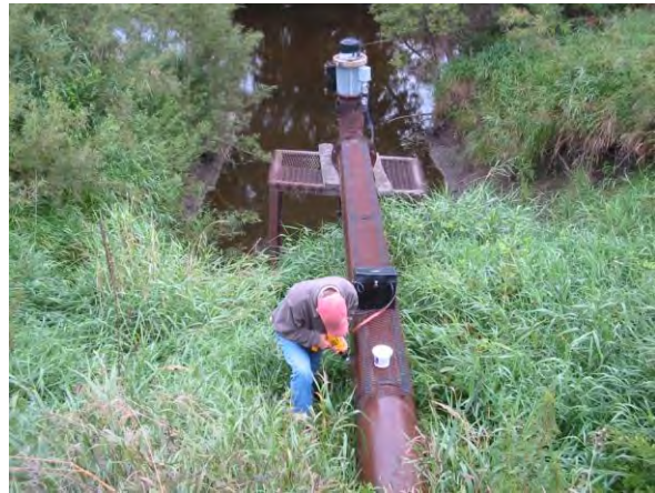
Measuring flow with doppler meter
