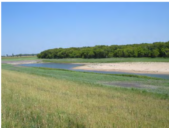
Borrow areas partially filled with runoff water
