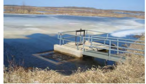
Gated Principal Outlet Structure
