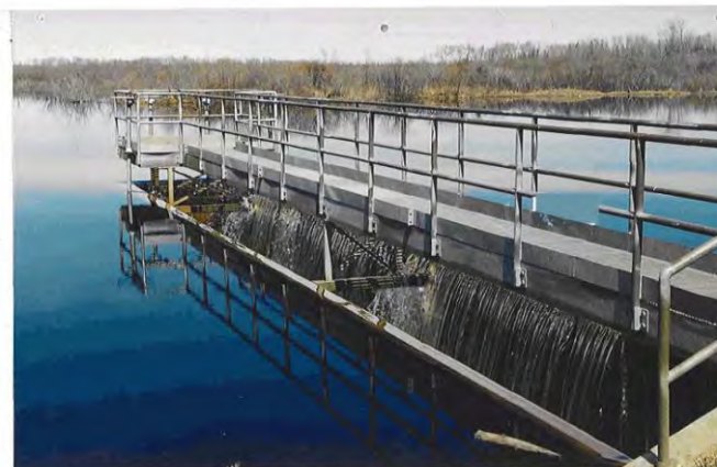
South Pool - Gated Principal Outlet Structure
