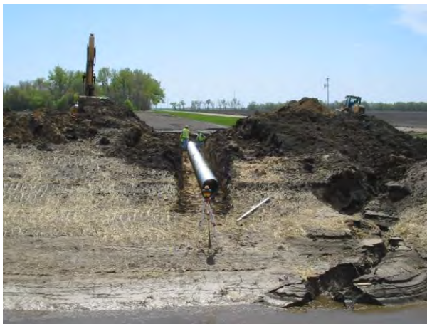
Installation of field drainage culvert
